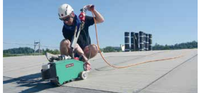
Flameless welding of modified bitumen with the BITUMAT B2.
