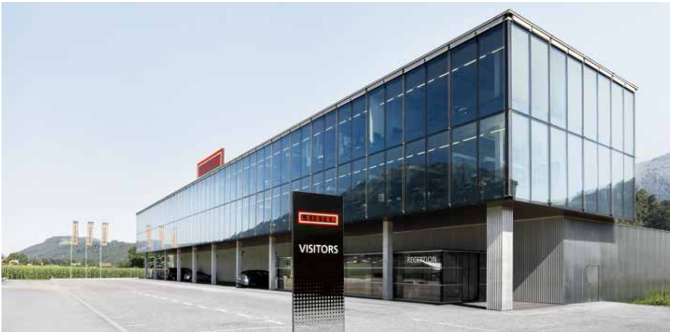
Leister AG, Headquarters, Kaegiswil, Switzerland
