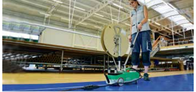
An economical, ergonomic tool for the welding of reinforcement tapes.
