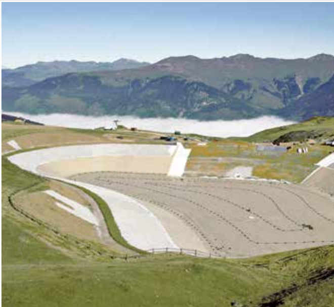
Water Reservoir, HDPE 0.08 inch (2 mm)
