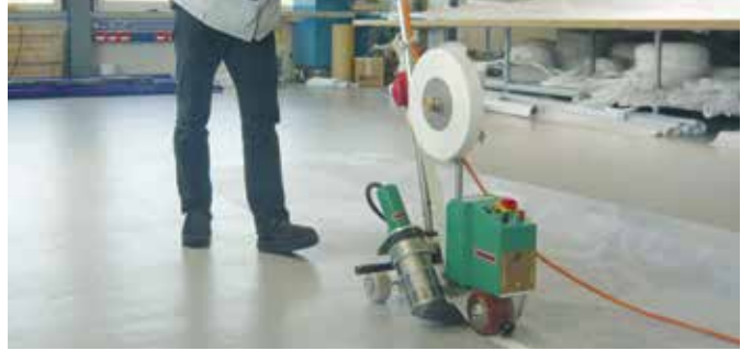
Welding tape at maximum speed.
