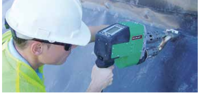
The powerful WELDPLAST S4 at work.
