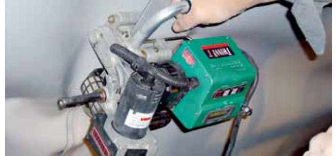
TWINNY T, with convenient cross-handle, at work overhead welding in a tunnel.
