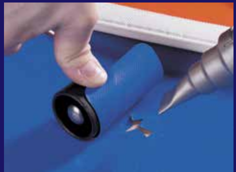
Welding patches or any other repair work
